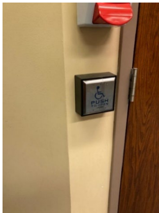
Photo 1: Accessible push button to open door
