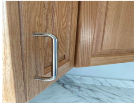
Photo 4: D-Pull handles on cabinets door
