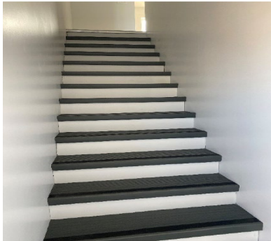
Photo 5: Contrasting colour on the rise and run of stairs
